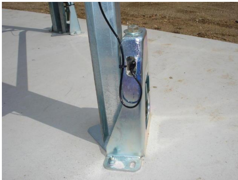
FIGURE 1: A FINISHED 'A' FRAME INSTALLATION
